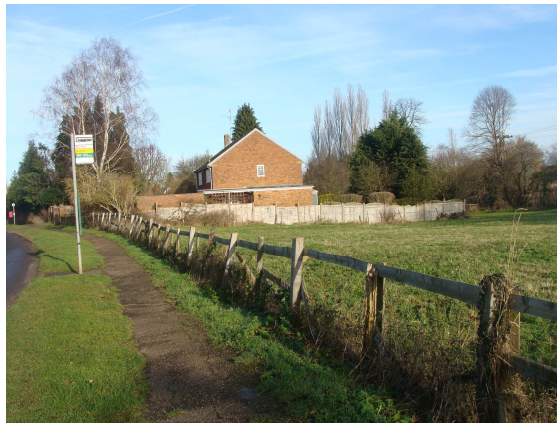
Picture 34 - Little Ash House and adjoining paddock to the south is proposed to be excluded from the Conservation Area.
