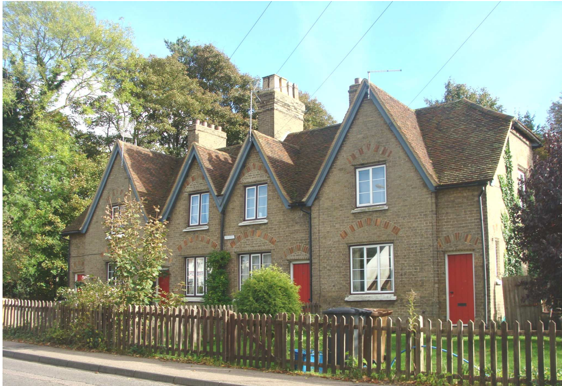
Picture 12. Gable Cottages, an important group of 19 th century properties that is important in the local street scene which should be retained.
