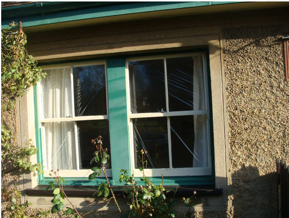
Picture 30 – Window detail of Smithy Cottage, built in 1936.
