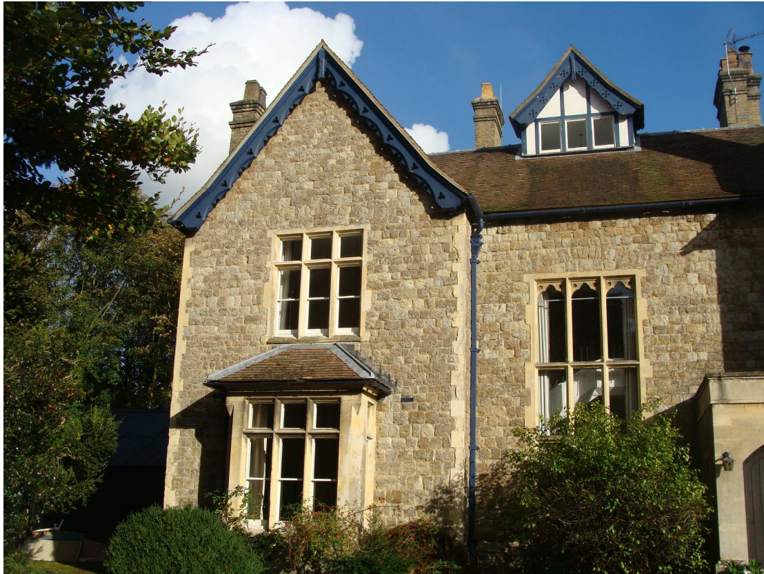
Picture 10. 19 th century former Vicarage for Rev H F Johnson. Designed by G E Pritchett.
