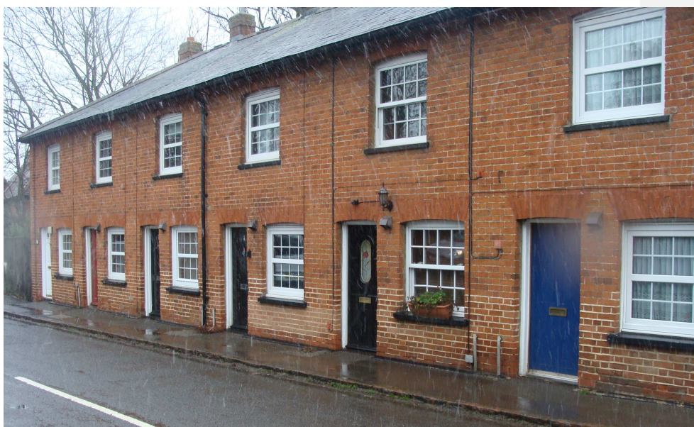
Picture 12 - Red Brick Cottages. Windows are modern replacements but because they are all similar they achieve an acceptable degree of architectural rhythm and unity.
