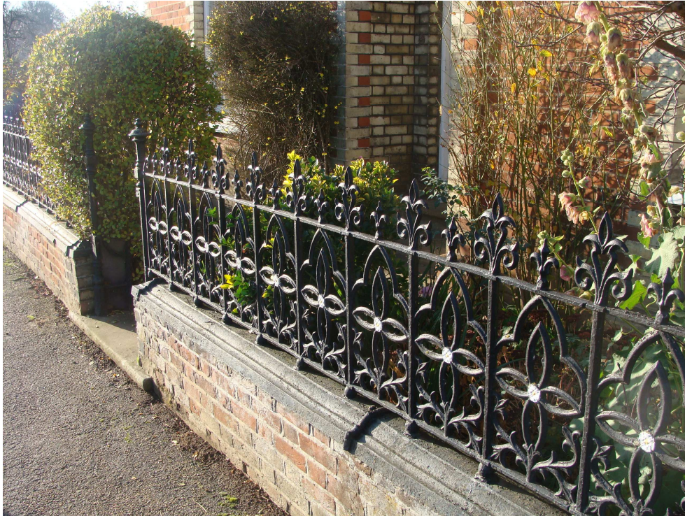
Picture 13 – attractive 19 th century railings to front of Ashford House.
