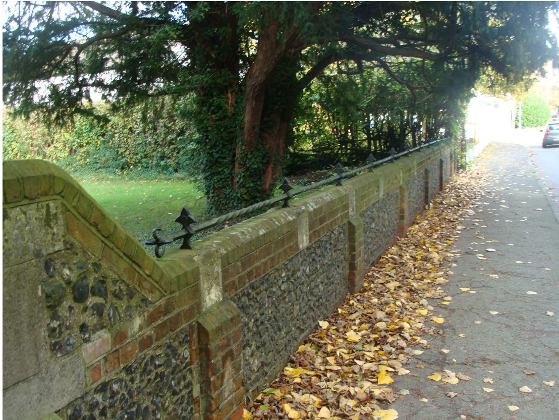
Pictures 7 and 8. Gate and fine 19 th century boundary wall to churchyard.
