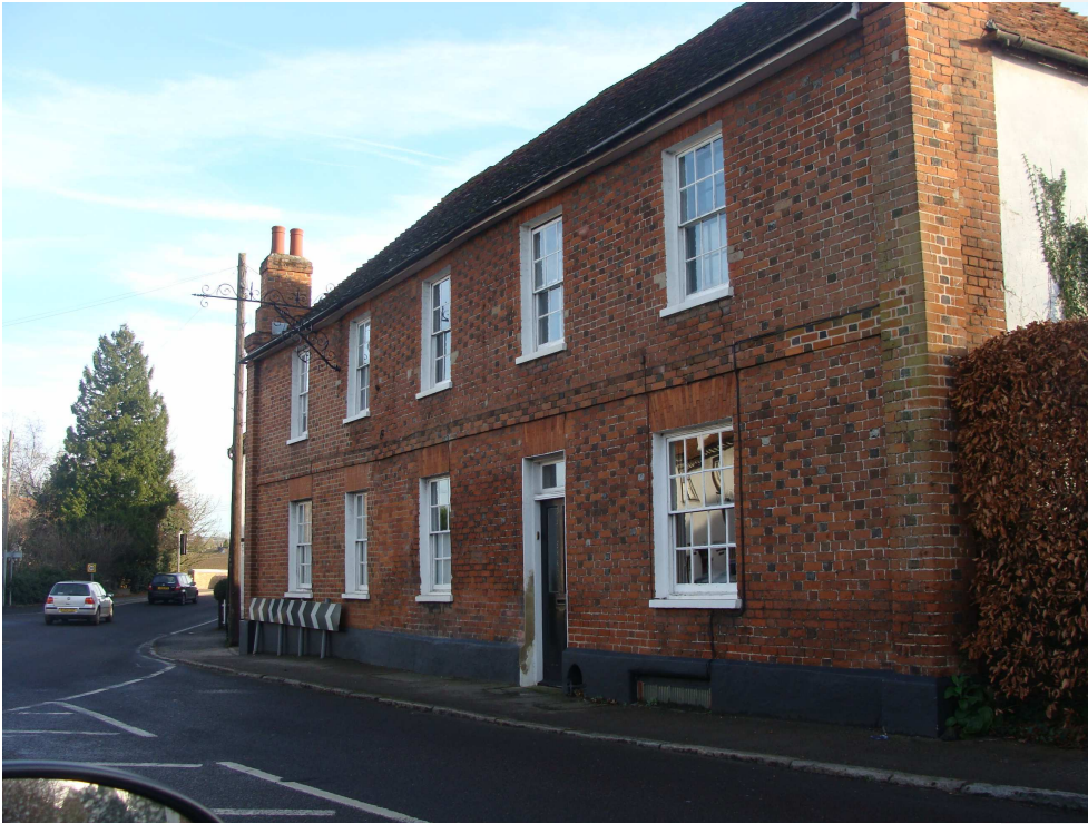
Picture 28 - The Angel, Stortford Road, a former inn. Probably 17 th in origin, listed grade II.
