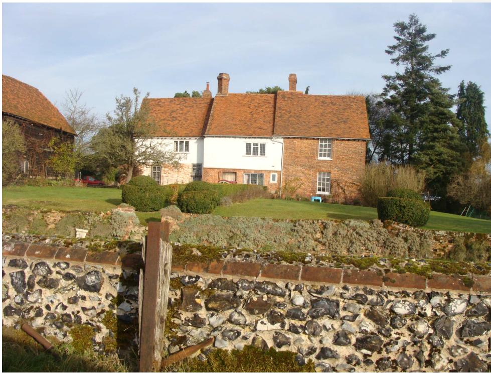
Picture 21 – Clintons, Grade II*. A fine early 15 th century timber frame and plastered hall-house at the centre of a group of historical buildings at this manorial site.
